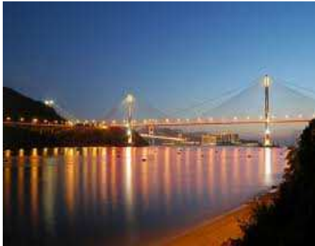
Ting Kau Bridge
